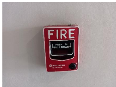
Fire Alarm Manual Station
